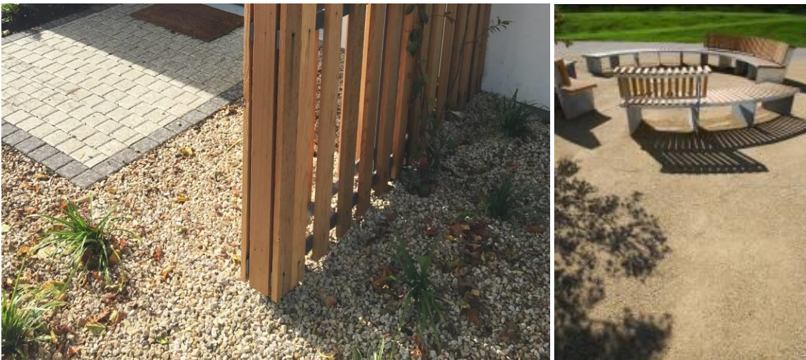
Figure 16: Range of hard landscape finish details (from left to right): permeable gravel detail, self-binding gravel.
