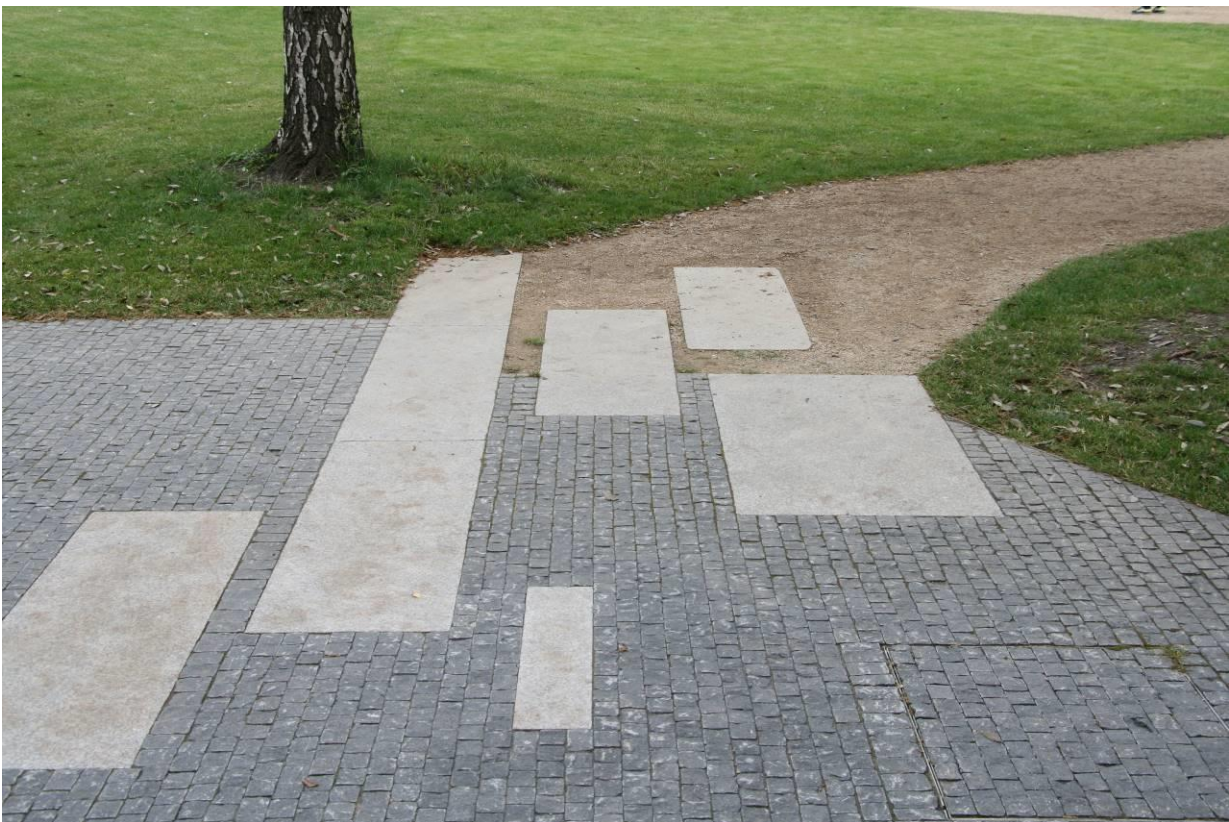
Figure 17: Mix of small and large format natural stone paving integrated with self-binding gravel.
